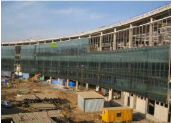
Curtain Walling Structure- Mumbai New Airport Terminal
