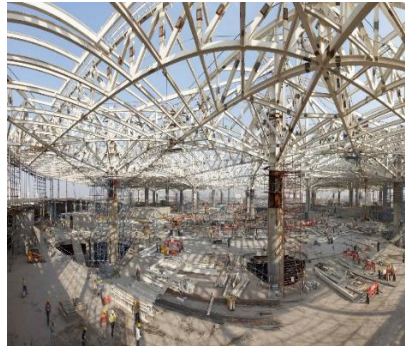
Curtain Walling Structure at Mumbai Int'l Airport
