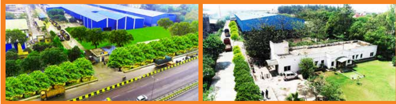
Sikandrabad, Uttar Pradesh (Unit-1 & Unit-2) Installed capacity of 2,55,000 MTPA
