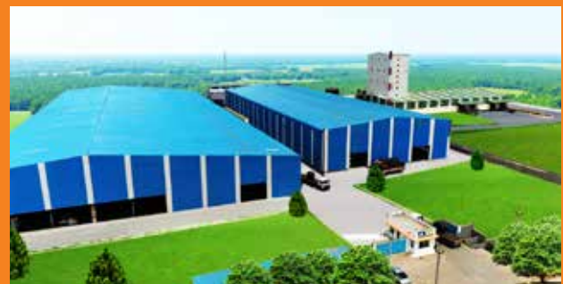
Hindupur, Andhra Pradesh Installed capacity of 1,20,000 MTPA
