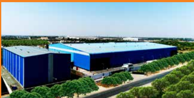
Sanand, Gujarat Installed capacity of 1,25,000 MTPA
