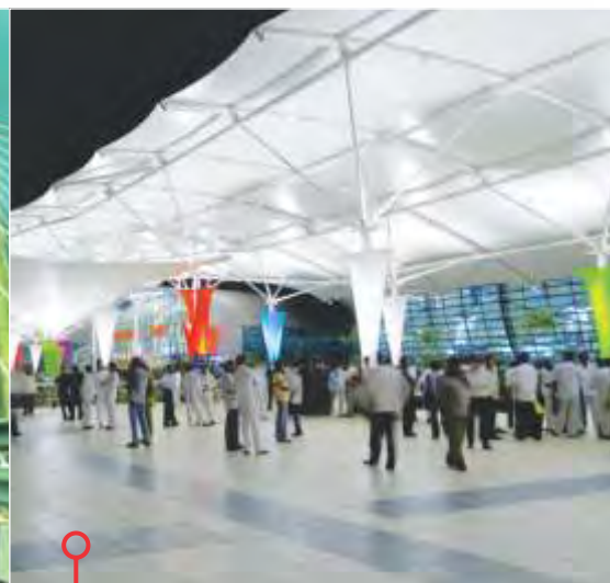
Tensile Membrane Structures- Mumbai Airport
